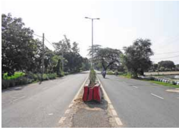
Road connecting towards Nizampur
