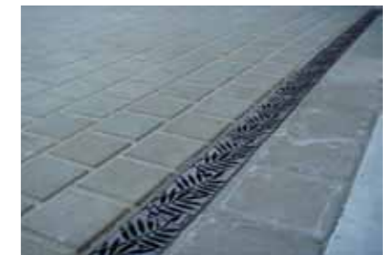
Road Section showing drain channel connection – Section BB'
